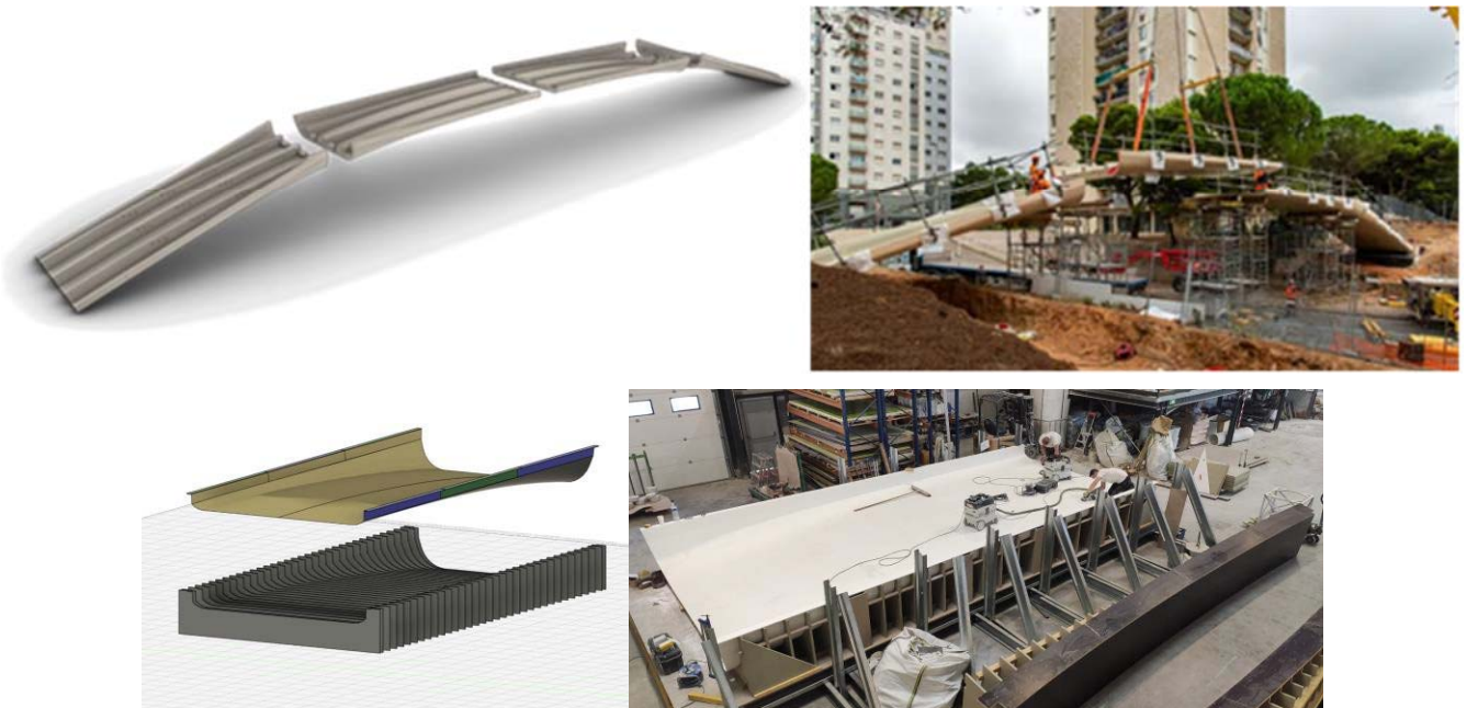
Figure 10. Main structure in 4 identical shells and unique formwork
